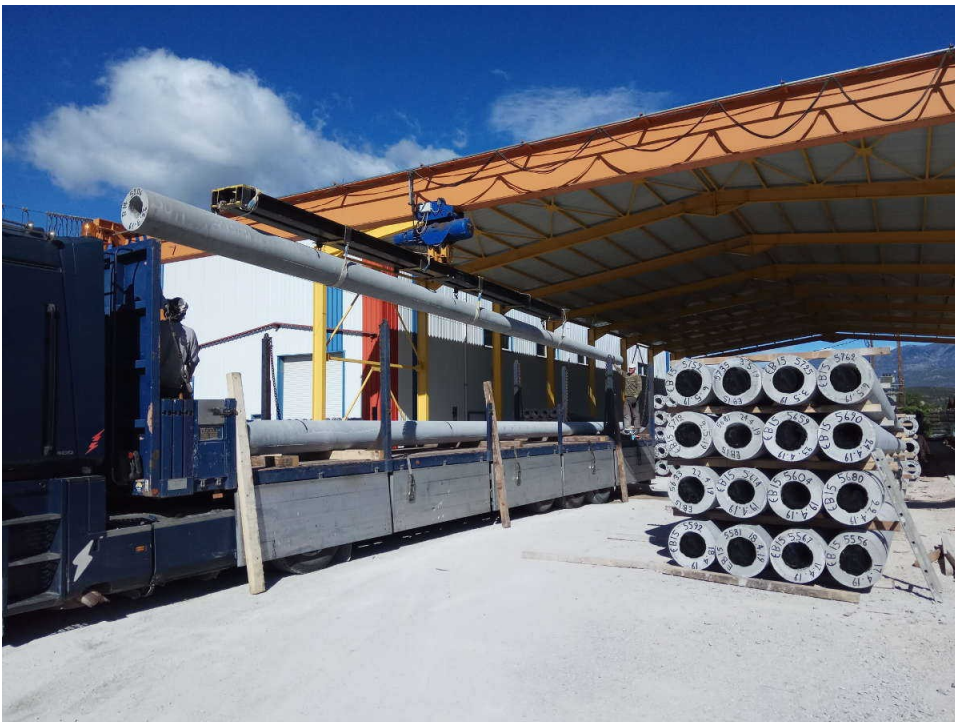
Pic. 6 Pole loading on truck
